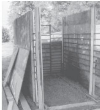
Covering a pickup livestock rack with plywood resulted in a tight little shed for storing lawn mowers and tools, says C.F. Marley.
