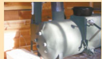
A heated anti-freeze mixture is pumped through 500 ft. of plastic tubing in the floors.
