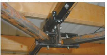
Metal bracket is attached to opener's chain and rides back and forth along the rail.
