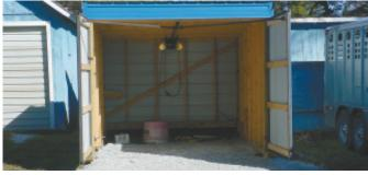
Glen Schweppe uses a single garage door opener to open a set of double doors on his home-built garage.
