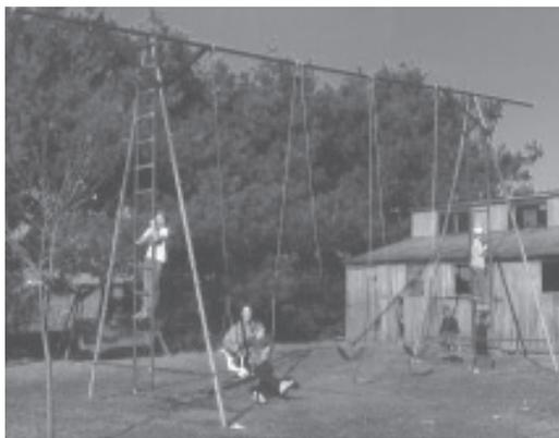
Gene Boehler built this 15-ft. high swing for his granddaughter, using 2 1/2-in. steel pipe for the top rail and 1 1/2-in. galvanized sq. tubing for the legs.
