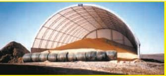
This is a simple solution to grain storage problems. My neighbor Robert Friest put up a 50 by 100-ft. hoop building to hold about 8,000 bu. of high-moisture shelled corn. One end of the building is enclosed. The other is blocked by a row of round
