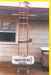
Hauling 50-lb. packs of roofing shingles up a ladder can be hard work. To make the job easier I use a hand-operated winch attached to a board on back of the ladder. Cable from the winch leads up to a pulley on the ladder is top rung, and then back down to an L-shaped wooden carrier with a hook on top of it. Four small metal trolleys on back of the carrier keep it from accidentally sliding off the side of the ladder.
