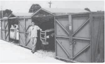
Charles Marley, St. Peters, Mo.: "Here's how I made a quickie shelter with no extra framing. I bought three shipping containers, which are readily available, and then bridged the spaces between them with sections of gable roofing.
