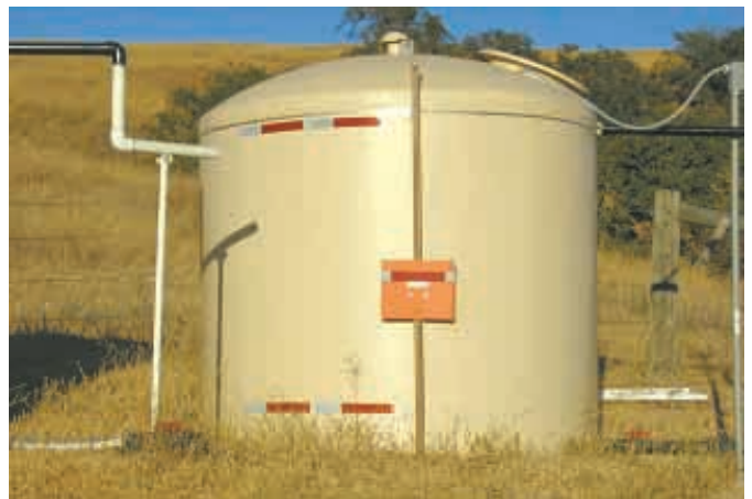
Ken Brading wanted to see the level on his two 2,150-gal. drinking water storage tanks, which sit about 700 ft. up a hill behind his house (right). So he fitted the tanks with float-style level indicators, and then put peel-and-stick reflector tape on them.
