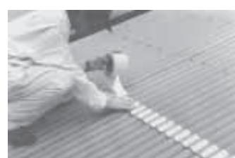
Peel & Seal roofing is an aluminum-backed, rubberized asphalt product that you simply roll out and stick in place.
