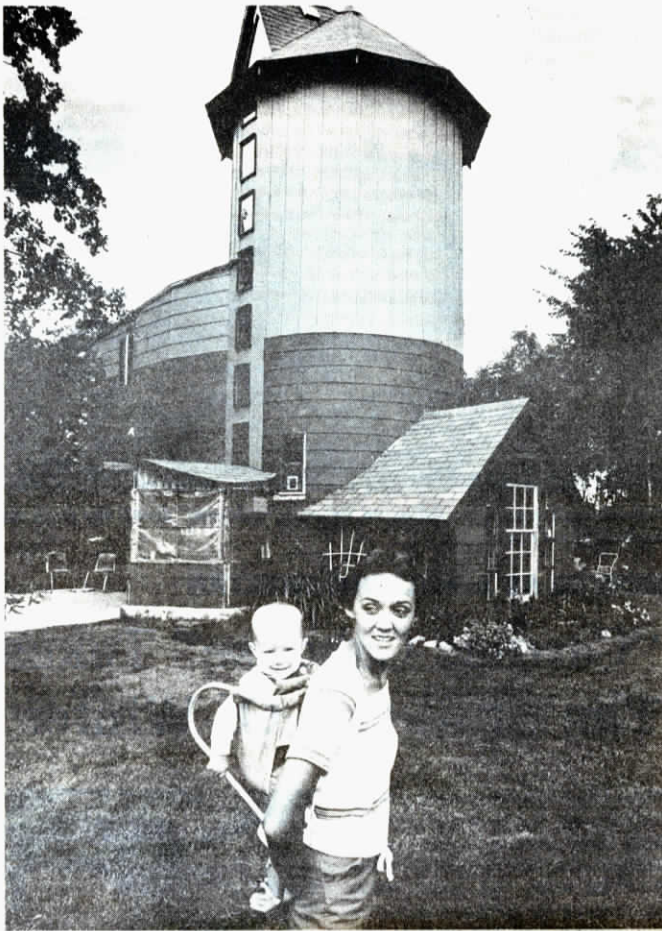
Lumber from a neighbor's hog barn was used on additions that surround Pat and Sharon Kennelly's silo home.
