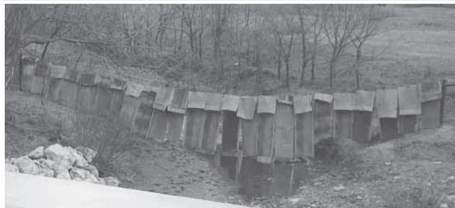
**Fence crossing consists of a series of corrugated barn roofing tin panels bent over a cable. Panels pivot backward as water rises, then fall back in place as water recedes.**
