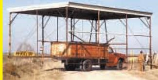
this car wash roof measuring 20 by 36 by 16 ft. tall using an old grain truck with a 16-ft. bed. He built a structure inside the truck box that held it up. He plans to build onto the sides of the roof to make a barn. **(Dava Carter)**
