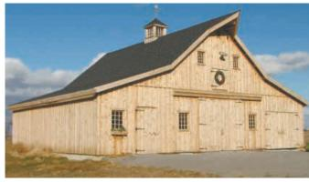
Len Dickinson offers barn kits based on historic post and beam timber framing methods. By varying roof pitches, eave lengths and other details, each building can be customized.
