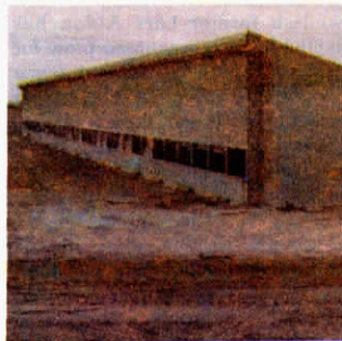
South-facing walls open automatically when sun comes up, close when it goes down at night.
