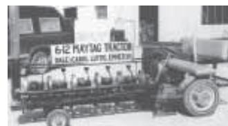
Luttig built a tractor powered by Maytags. The motors are timed to run at the same speed.
