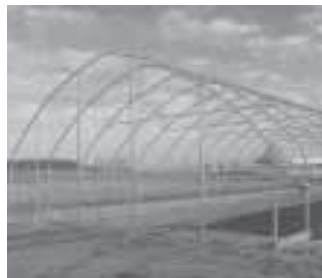
Cold frame shell is made of square tubing (left). Besides shedding snow, the arch reduces condensation build-up and water dripping inside.
