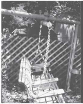
A pivot is welded to the frame and attached to a smaller 2-in, horizontal pipe, which has chains attached to swing.
