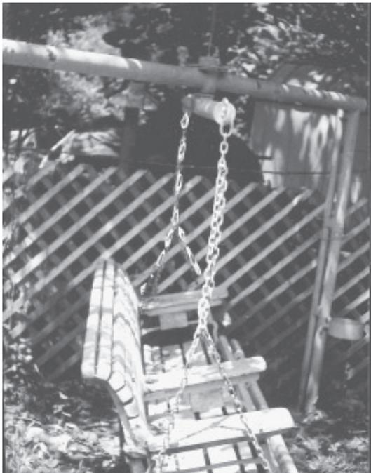
A pivot is welded to the frame and attached to a smaller 2-in. horizontal pipe, which has chains attached to swing.
