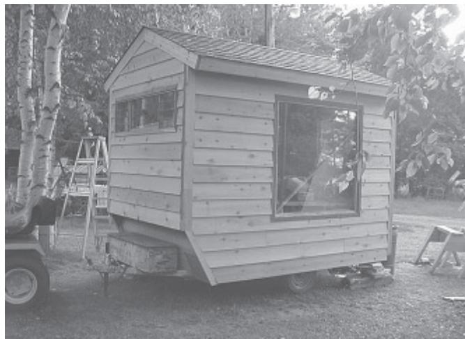
Loren Etter built this insulated wooden shack on the frame of a 2-wheeled trailer. He tows the portable shack behind his garden tractor.
