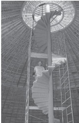
Access from the first floor all the way to the cupola is gained by climbing a freestanding, 66-step circular staircase.
