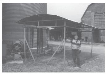
$\label{thm:continuous} \begin{tabular}{ll} Hubert Smith used sections of a damaged 3,000-bu. bin to make this car port. It measures 12 ft. wide by 22 ft. long and mounts on steel runners. \end{tabular}$
