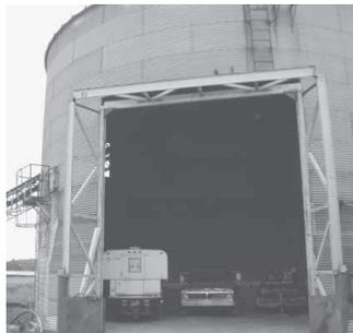
They cut a 20-sq. ft. hole in one side of bin and framed in a doorway with heavy steel trusses.
