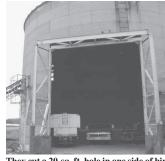
They cut a 20-sq. ft. hole in one side of bin and framed in a doorway with heavy steel trusses.
