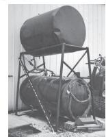
When the storage drum inside is full, oil is pumped to a pair of 300-gal. storage tanks outside the shop.
