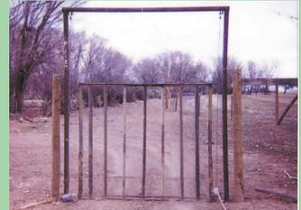
Weights connected to gate panel pull it back into full upright position.
