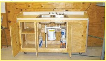
"Sink on wheels" is complete with a mini hot water heater. It can be moved around cattle processing barn as needed.
