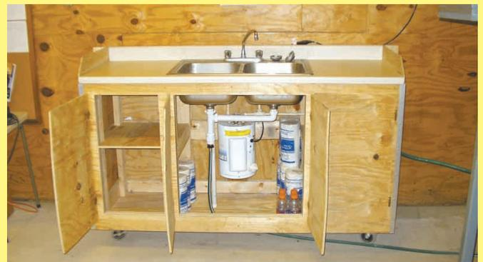
"Sink on wheels" is complete with a mini hot water heater. It can be moved around cattle processing barn as needed.
