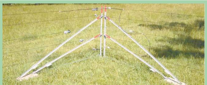
Speed Brace locks an angled T-post to any upright T-post to form a strong brace.
