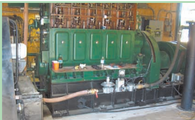
Process involves gasifying wood and other organic material and burning the gas in big engine-powered generators.
