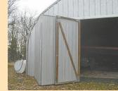
Tri-fold doors slide on a pair of conventional barn tracks, with each track covering two doors. The two inside doors are hinged and swing out.
