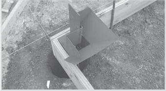
Metal bracket screws onto building's splash board.
