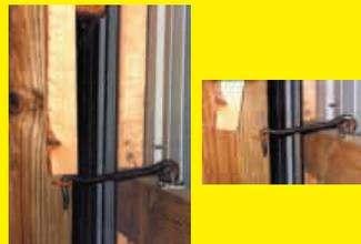
door. Rather than replace the lock, I decided to make my own lock. I simply installed a large hook and eye with a pivoting piece of wood above it that holds the hook in place. No one can shake it loose by rattling the door, and I can release the hook easily by pivoting the wood to the side. **(Allen Beiler, New Holland, Penn.)**
