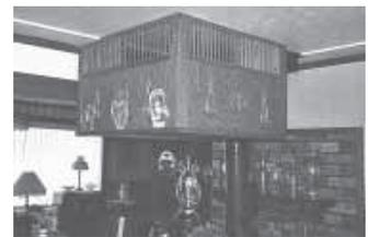
A copper box, mounted inside a wooden enclosure on the ceiling, collects heat from top of stove and blows it into ductwork. The temperature can be 69 degrees, yet the stove can heat the house back up to 74 degrees in only about two hours," says Mahowald. "It took me three winters to figure out how to get the right combination of coils, relays, and temperature sensing units to coordinate with the furnace fan.
