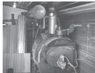
The water jacket simply wraps around the flue and is plumbed into the boiler.
