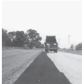
Add-on box can be used to deliver gravel as well as hot and cold asphalt.
