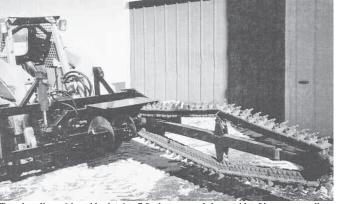
Trencher digs a 6-in. wide slot 6 to 7 ft. deep around the outside of basement walls to relieve the inward pressure on buckled basement walls.
