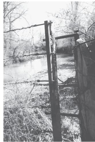
A piece of 3/8-in. threaded rod connects to the end of each fence wire for easy tightening with a wrench.
