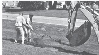
Walking plow hooks up to backhoe bucket on back of a tractor.
