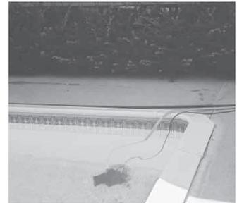
A submerged pump circulates water through the solar heated hose.
