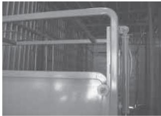
Cast steel and aluminum elbows make it easier to put right angles on square tubing.
