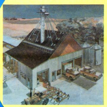
Cube-style overhead bins are filled the same as conventional bins by auger or bucket elevator. But, for moving material out, gravity takes over.
