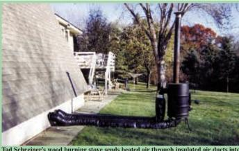
Tad Schreiner's wood burning stove sends heated air through insulated air ducts into his shop, which is located under the living space in his house.
