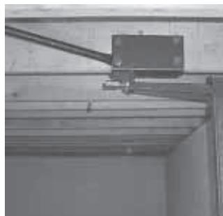
Threaded rod on joist bracket pushes out against wall brace.
