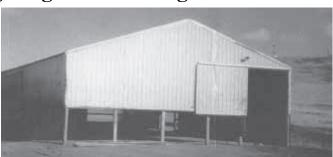
Weiss adds height to building after it's been braced for transport. He uses a series of hydraulic jacks to raise it up.
