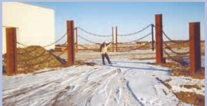
Massive gate was made using a large chain from an old oilfield dragline. It has 6-in. links.
