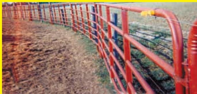
When we put metal cattle panels up in our corral, we needed a way to attach insulators to the top of the panels in order to power an electric fence at the other side of the lot. To attach the insulators, we put Velcro patches on the pipe and also on the insulators. Then we stuck the
