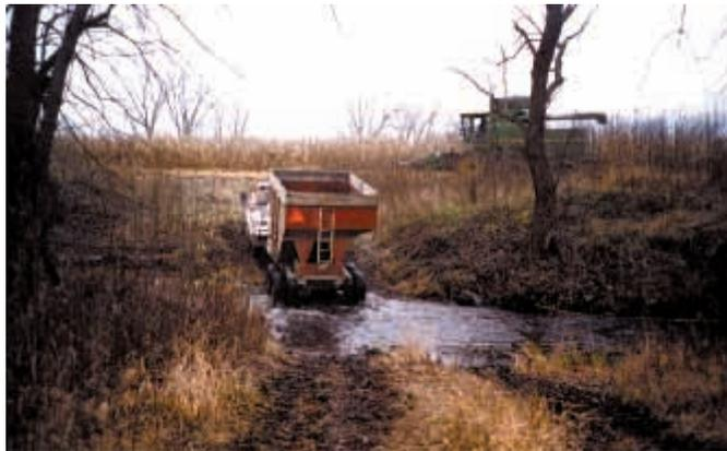
Sloped cut through creek banks angles down through water. Sides of creek bank and creek bottom are underlaid with rocks so Phillips can drive through without sinking in.
