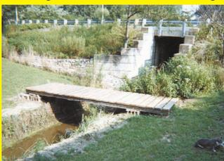
a 12-ft. high pile of wood for just \$25. It consisted of 2 by 6's, 8's, and 10's in 3, 4, 5, and 6-ft. lengths. I used some old 6 by 6 treated posts for runners under the bridge. The two bridges cost a total of only about \$10. Each bridge can hold about 2,500 lbs., which is enough to sup-
