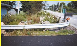
the highway contractor for \$90. I tied into the guard rail with a 90 degree section that runs into my driveway to protect my house. Then I placed several big boulders - 35 tons worth - behind the guard rail. Now if someone accidentally drives anything less than an Abrams tank into my yard, he'll come off second best.
