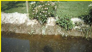
digging into the banks and kicking up debris. Occasionally it would overflow, creating a small lake that lapped up to my house. I dug it out and then lined it with used chain link fence in order to keep muskrats from digging into the banks. No more muskrat problems.
