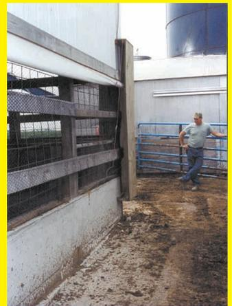
I regulate air flow in my cattle building using a rolling curtain. The curtain is prevented from flopping around by boxes at the corner. As the curtain is rolled up or down, a rod running through the bottom is held snugly in place by the boxed-in corners. **(Charles Kruegel, Shoboiner, Ill. 62885).**
