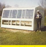
Here are a couple pictures of a greenhouse I built. I had been saving glass from various sources for many years and finally figured out something to use it all for. I used all treated lumber and built the greenhouse on 4 by 4 skids so it can be easily moved, if needed.
