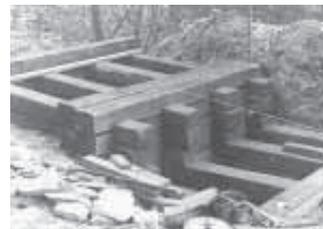
Railroad tie footings, laid log cabin-style at each end of the bridge, provide solid support.
