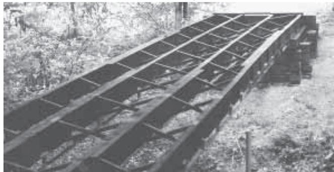
John Slywczak used beams from a 52-ft. trailer to make a bridge that crosses a stream on his farm.
